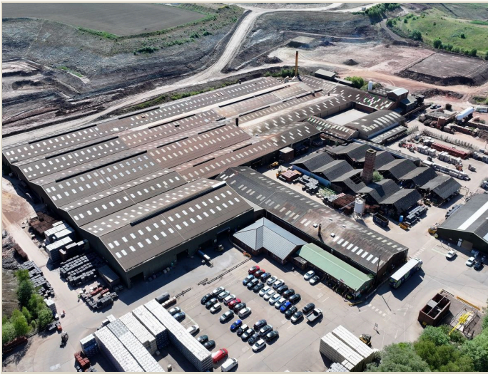
FULL SITE PHOTO
