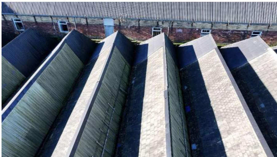
FIGURE 18: AERIAL PERSPECTIVE OF ROOF 18
