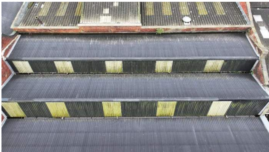
FIGURE 10: AERIAL PERSPECTIVE OF ROOF 10
