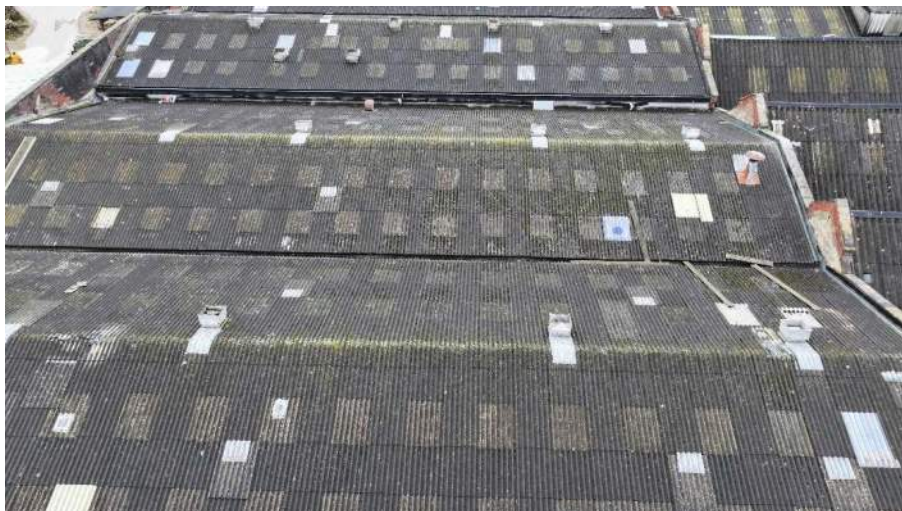
FIGURE 3: AERIAL PERSPECTIVE OF ROOF 3
