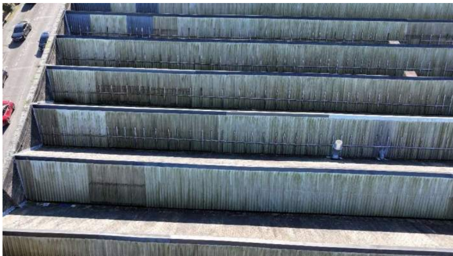
FIGURE 16: AERIAL PERSPECTIVE OF ROOF 16
