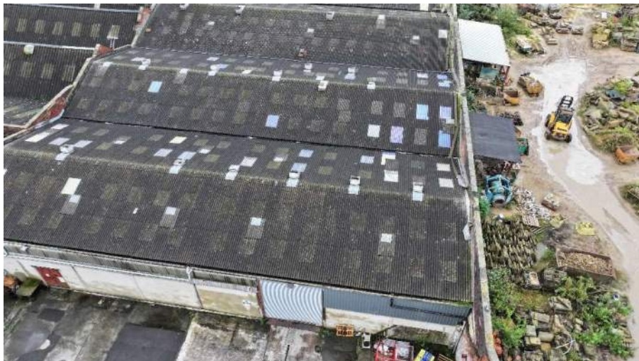
FIGURE 1: AERIAL PERSPECTIVE OF ROOF 1
