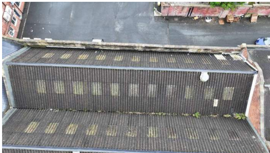
FIGURE 5: AERIAL PERSPECTIVE OF ROOF 5
