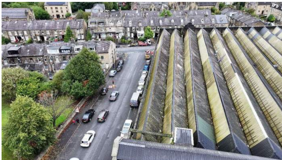
FIGURE 15: AERIAL PERSPECTIVE OF ROOF 15
