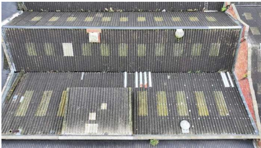
FIGURE 9: AERIAL PERSPECTIVE OF ROOF 9
