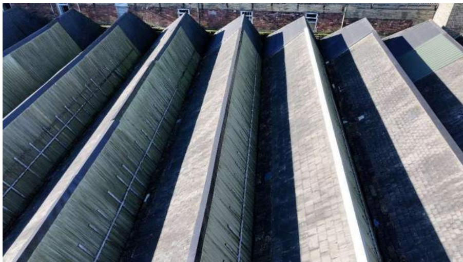
FIGURE 17: AERIAL PERSPECTIVE OF ROOF 17
