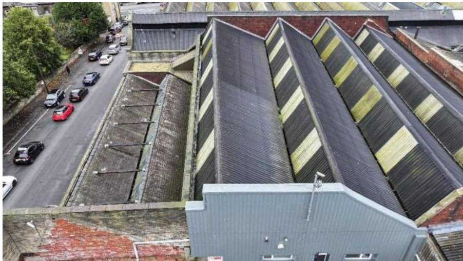
FIGURE 11: AERIAL PERSPECTIVE OF ROOF 11
