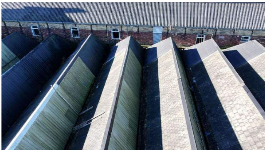
FIGURE 19: AERIAL PERSPECTIVE OF ROOF 19
