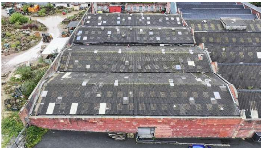
FIGURE 4: AERIAL PERSPECTIVE OF ROOF 4
