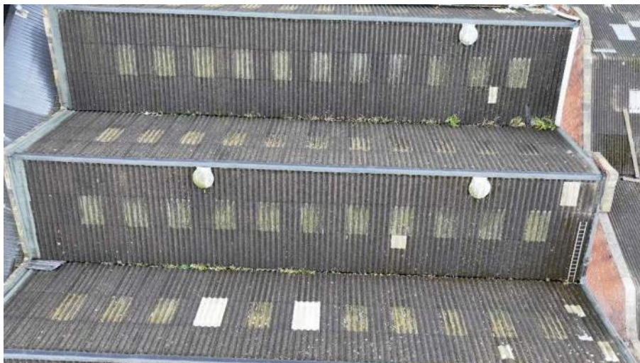
FIGURE 6: AERIAL PERSPECTIVE OF ROOF 6
