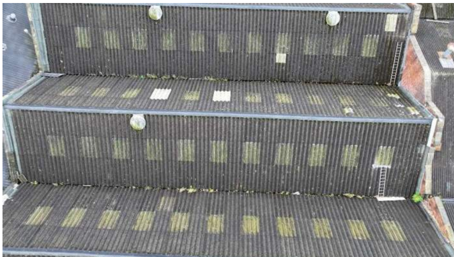
FIGURE 7: AERIAL PERSPECTIVE OF ROOF 7
