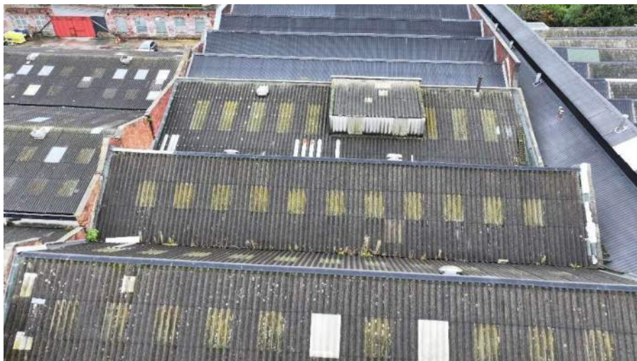
FIGURE 8: AERIAL PERSPECTIVE OF ROOF 8
