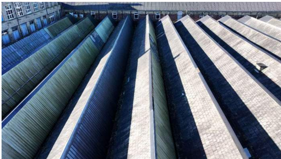
FIGURE 20: AERIAL PERSPECTIVE OF ROOF 20
