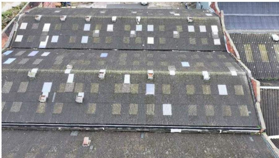
FIGURE 2: AERIAL PERSPECTIVE OF ROOF 2
